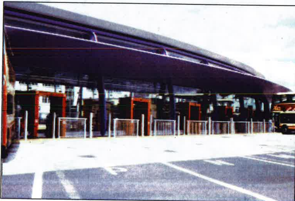
Figure 2.7: Burnley bus station bus departure bays
